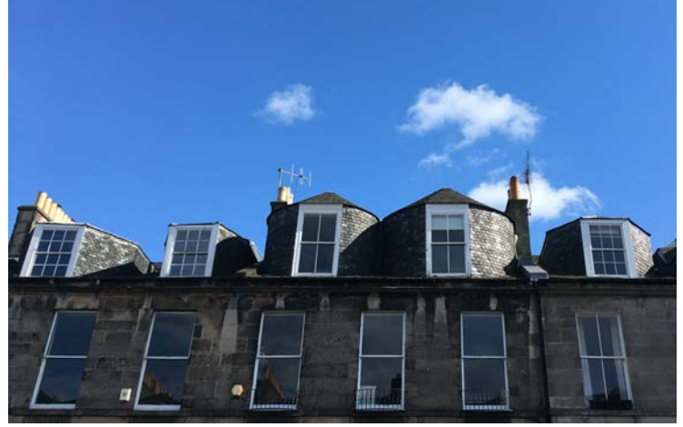
Design Statement 3e, Albany Street front view turret and bay window dormer formations
