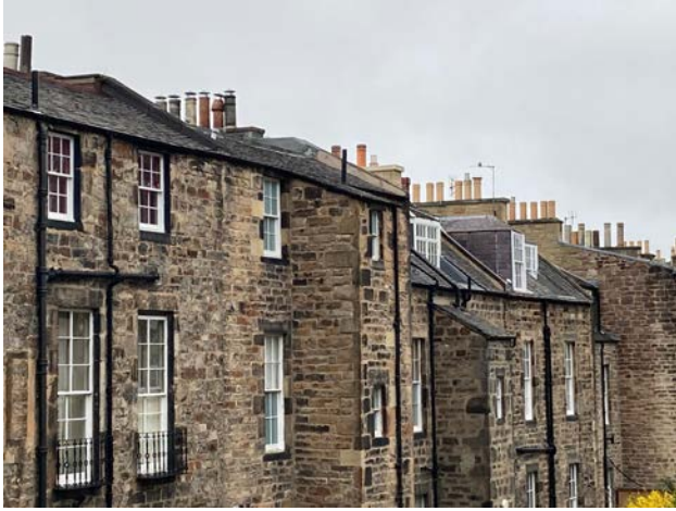
View B, Albany Street rear view, from Dublin Street Lane
