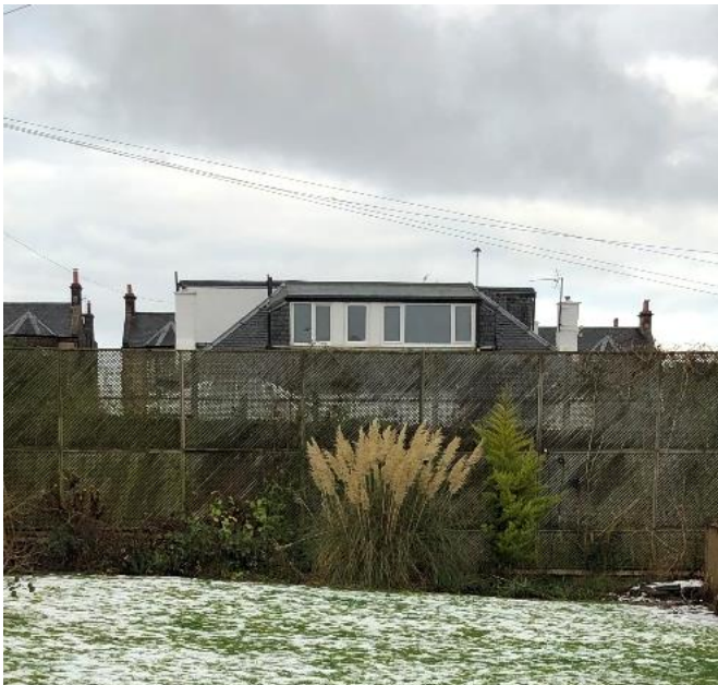
19a Hillhouse Road – rear of application site
