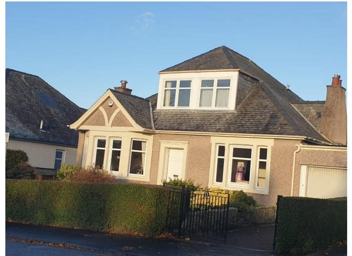
33 Orchard Road South (Principal Elevation)
