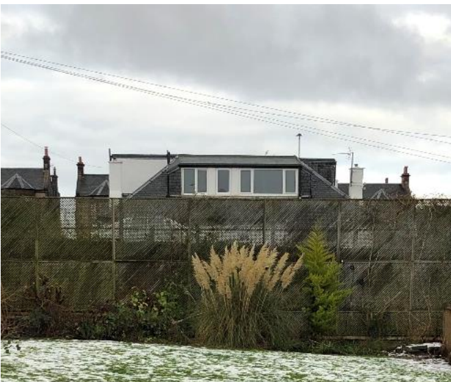
19a Hillhouse Road – rear of application site
