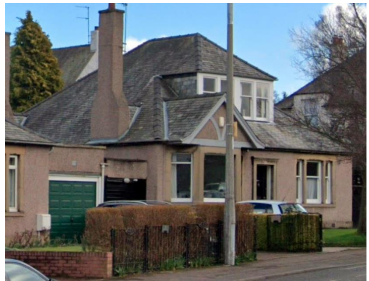
37 Orchard Road South (Principal Elevation)
